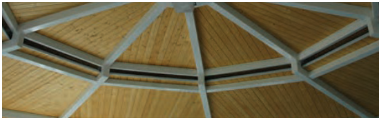
Interior view of Vented roof option
